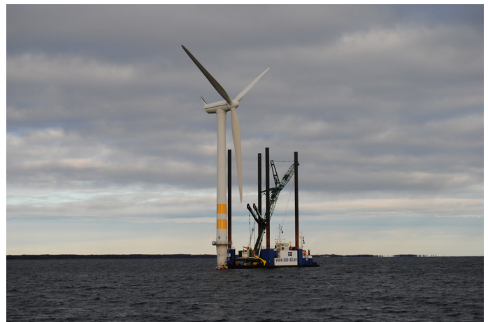
Specialized wind turbine technicians from Connected Wind Services were put at work when the Swedish wind farm Yttre Stengrund in Kalmar Sound was decommissioned as the first offshore wind farm in the World.
